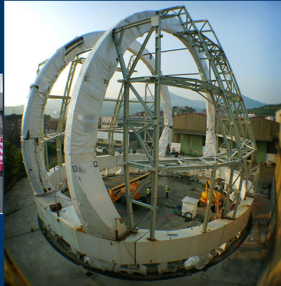
Factory Assembly in Bilbao, Spain (July, 2013)
